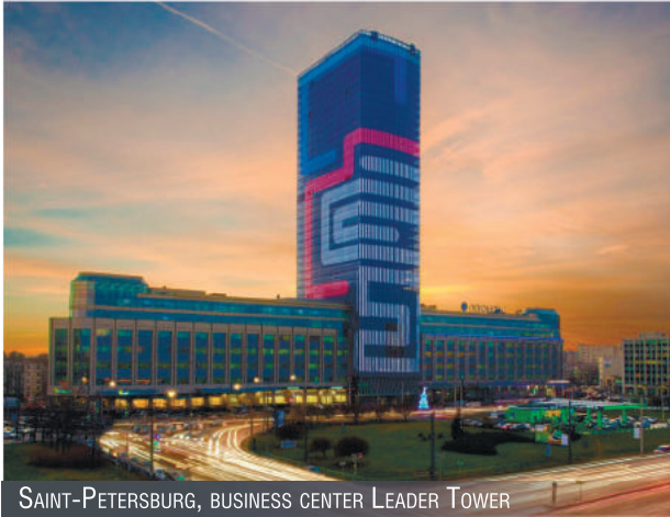
SAINT-PETERSBURG, BUSINESS CENTER LEADER TOWER
