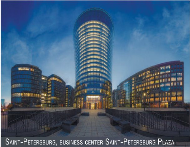
SAINT-PETERSBURG, BUSINESS CENTER SAINT-PETERSBURG PLAZA
